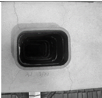
Clay Tile Liner Flue
