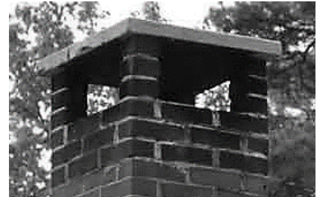
Concrete Cap Chimney Top
